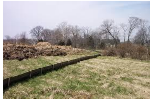
Geotextile silt barriers to be erected prior to earthworks commencing
