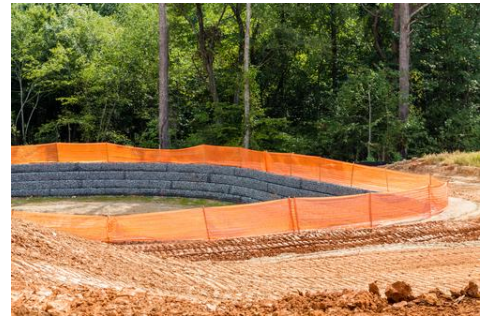
A settlement tank for holding silt contaminated water.
